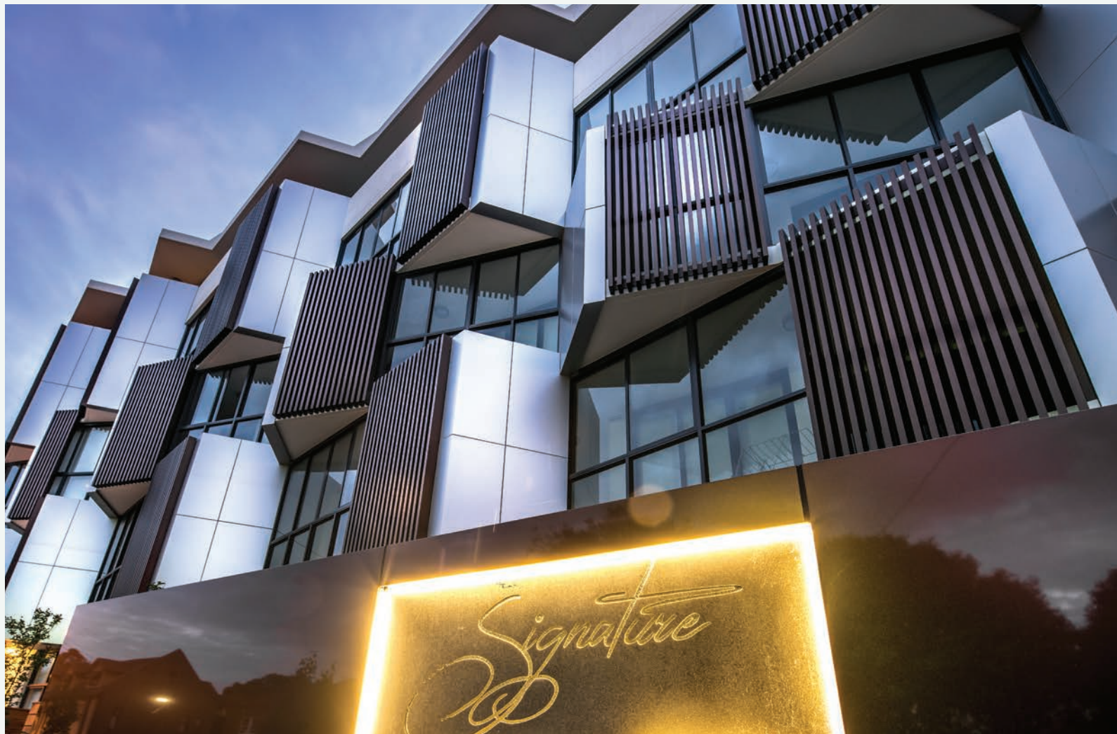
Signature Apartments, Ashfield 50 residential units
