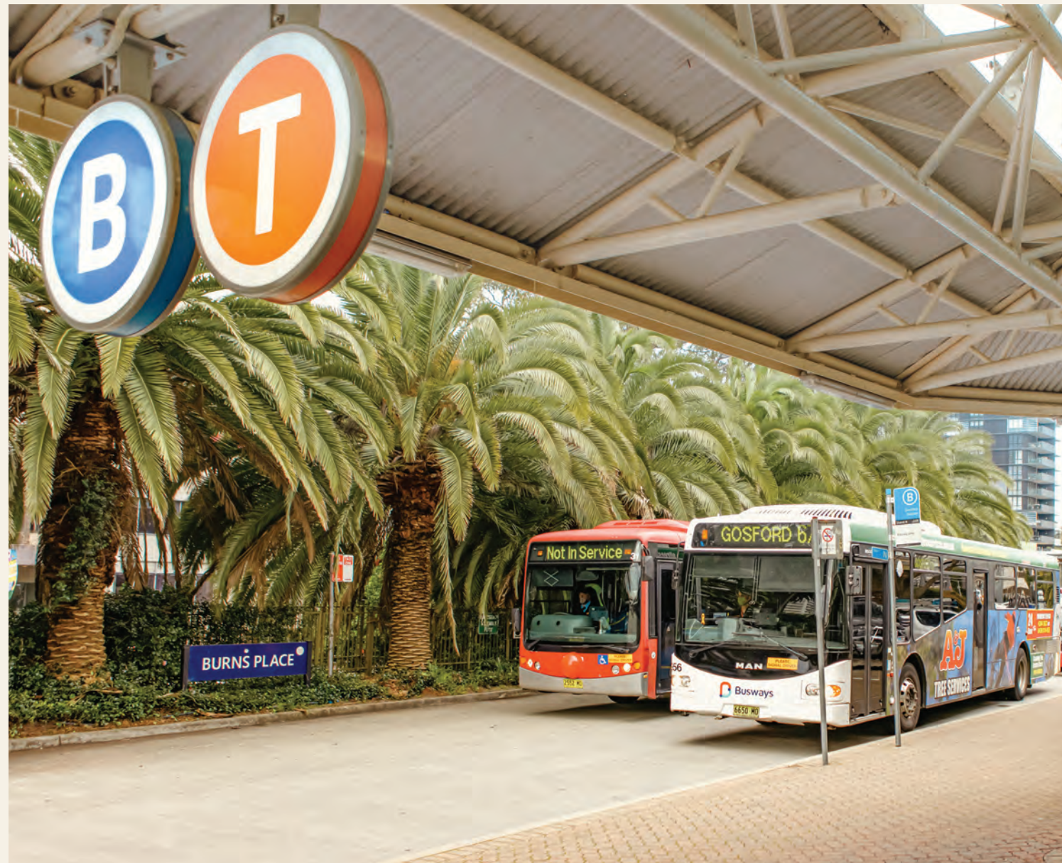
GOSFORD STATION AND BUS INTERCHANGE
